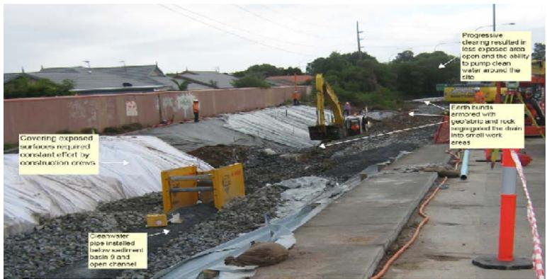
Figure 2. Construction of the 'triple-stack' design. Progressive clearing, segmentation, surface protection and clean water pipe construction.
