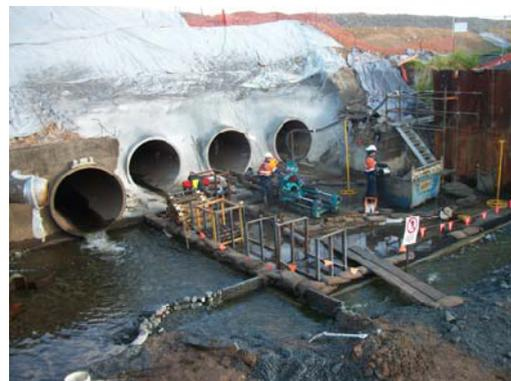
Figure 6. Clean water managed through work area to downstream during Kimberley culvert works.
