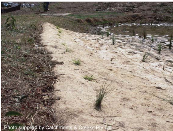
Photo 1 – Anchorage of the up-slope edge of an erosion control blanket
