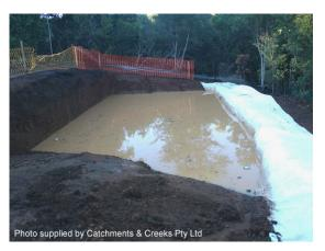
Photo 13 – Fully recessed basin with natural ground forming the spillway
