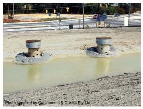
Photo 5 - Riser pipes under construction
