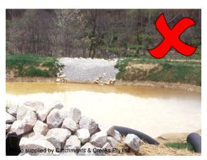
Photo 16 - Spillway crest with inadequate depth or profile
