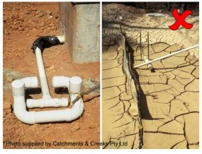
Photo 8 – Skimmer pipes must be protected from sediment build-up
