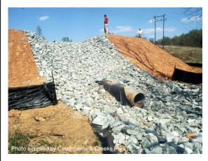
Photo 11 – Emergency spillway located within the fill embankment
