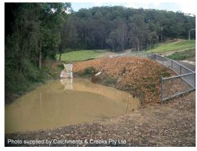
Photo 18 – Sediment basin with poor access for de-silting operations
