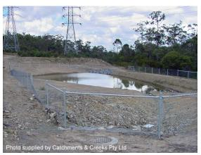
Photo 19 - Temporary fencing of a construction site sediment basin
