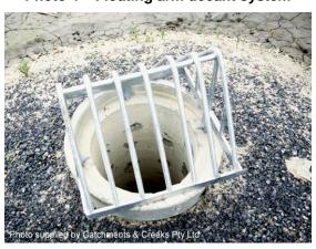
Photo 6 - Riser pipe with aggregate filter
