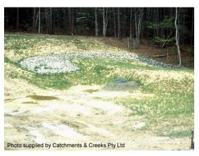
Photo 12 - Emergency spillway located within virgin soil to the side of the embankment
