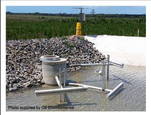
Photo 3 – Type A decant at low water level
