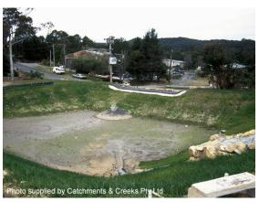
Photo 14 - Rock-lined spillway—note concrete sealing of the spillway crest
