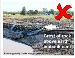
Photo 15 – Spillway rock protection sits above the embankment height
